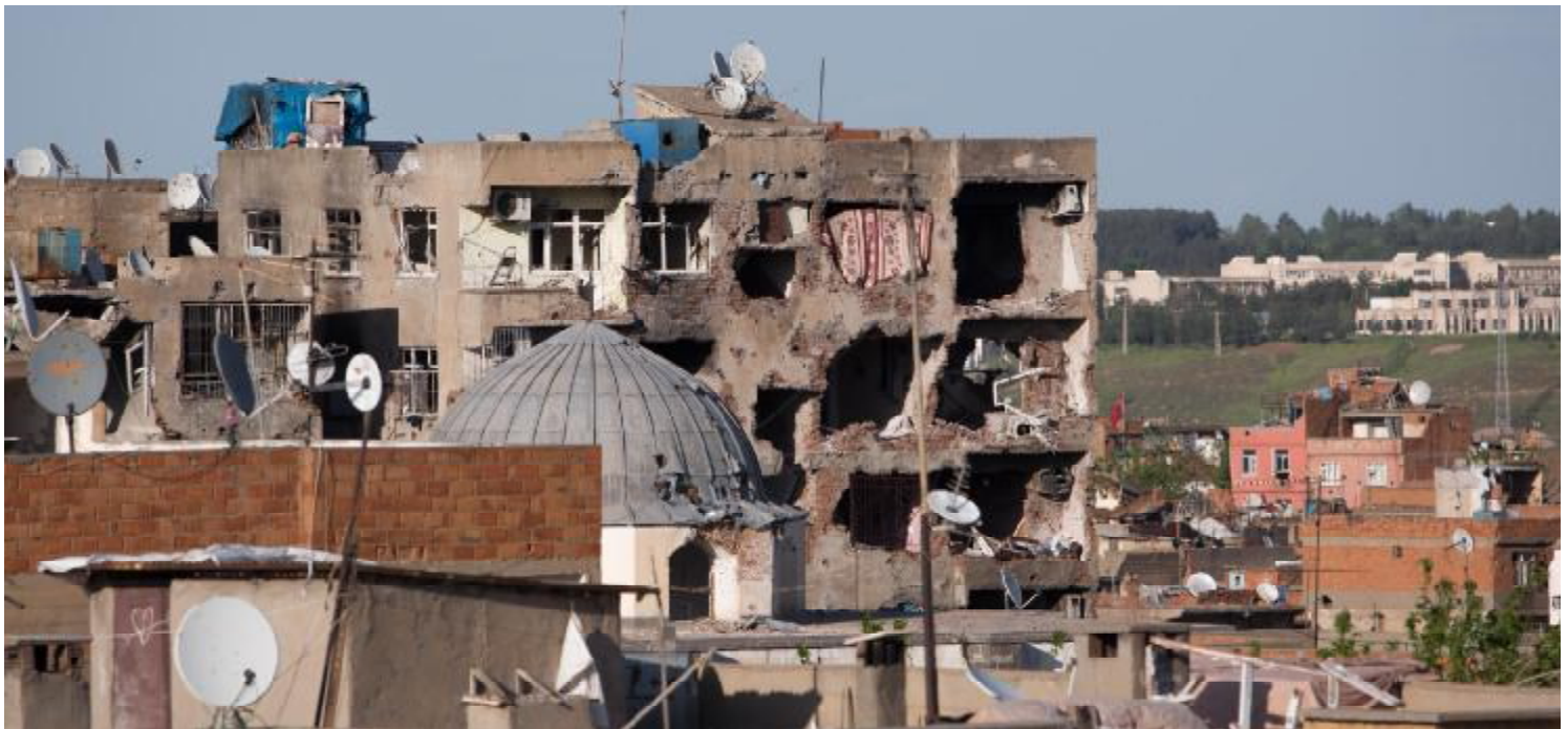
Heavily damaged building in Diyarbakir, Turkey, April 2016 after months-long army assault.
